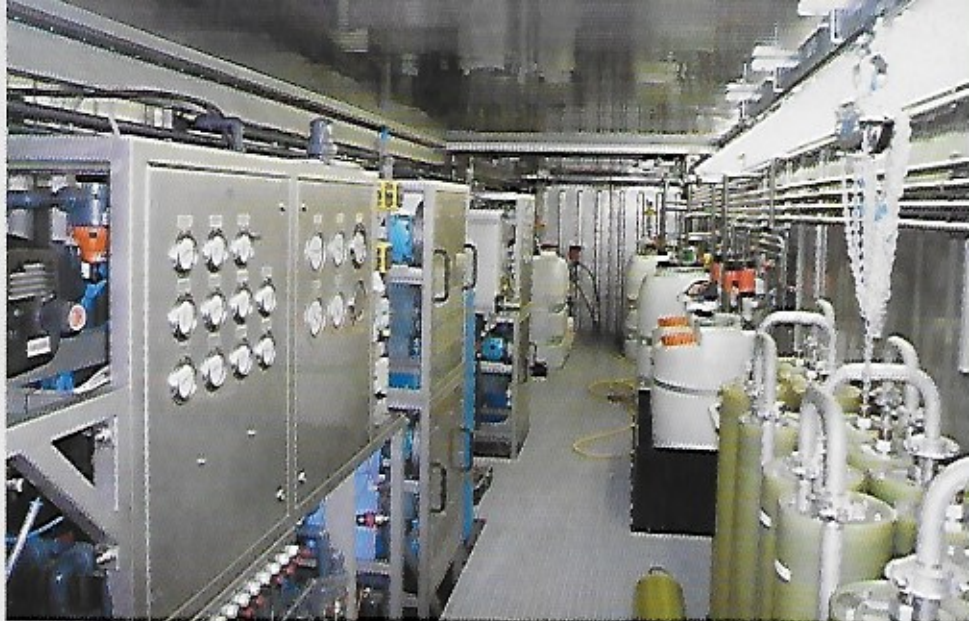
Left: Three parallel 70,000 gpd RO leachate treatment skids; right: 25,000-gcd containerized RO leachate treatment system
