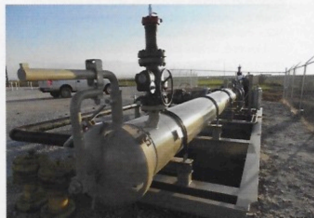
Figure 2. Designing pipelines for easy insertion and removal of pigs helps facilitate removal of liquids in the line. Photo courtesy of WeldFit Energy Group.
