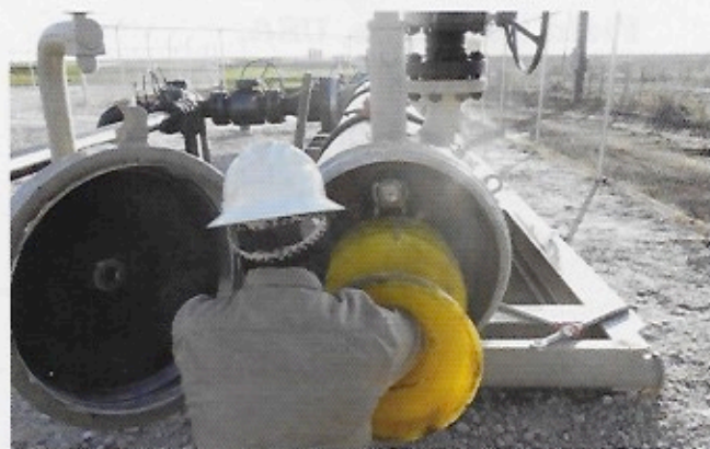
Figure 1. Pigs in an automated insertion system are lined up to be inserted on a schedule or as required. Photo courtesy of WeldFit Energy Group.
